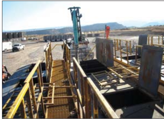
Equipment positioned in place to vacuum out a frac tank. Photograph courtesy of RAMVAC.
